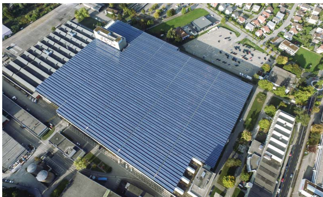
Zuchwil, Riverside solar power plant, completed in 2015
