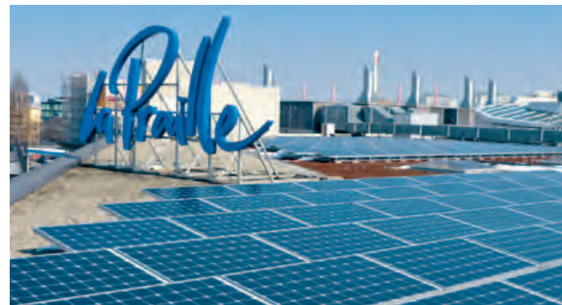
The pilot project generates roughly 177 000 kilowatt hours annually.
